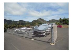
Based on "Full" Reserve Study by Association Reserves Hawaii LLC for period beginning January 01, 2011: Approx. 320 LF @ \$14,944 to \$19,840 (= approx. \$47/LF to \$62 LF) The fence is in fair to poor unsturdy condition. Several poles are rusted through at the base. The mesh is rusted and sagging. The intersect with the block wall has been damaged compromising the security of the boat storage.
