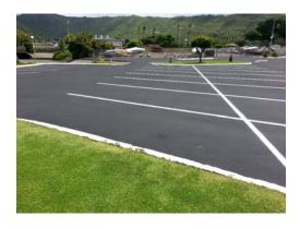
"Full" Reserve Study by Association Reserves Hawaii LLC for period beginning January 01, 2011: Parking lot & boat storage areas. The surface shows drying and some minor cracking and roughness. Curbs need repair. Seal coat is needed to extend the life of the asphalt and curbs.
